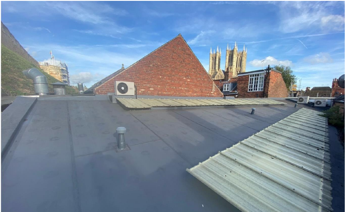
Photo of existing roof, showing existing air conditioning units
